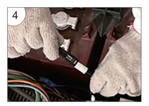
7. Connect the OBC bypass wire to the negative terminal of the battery.
